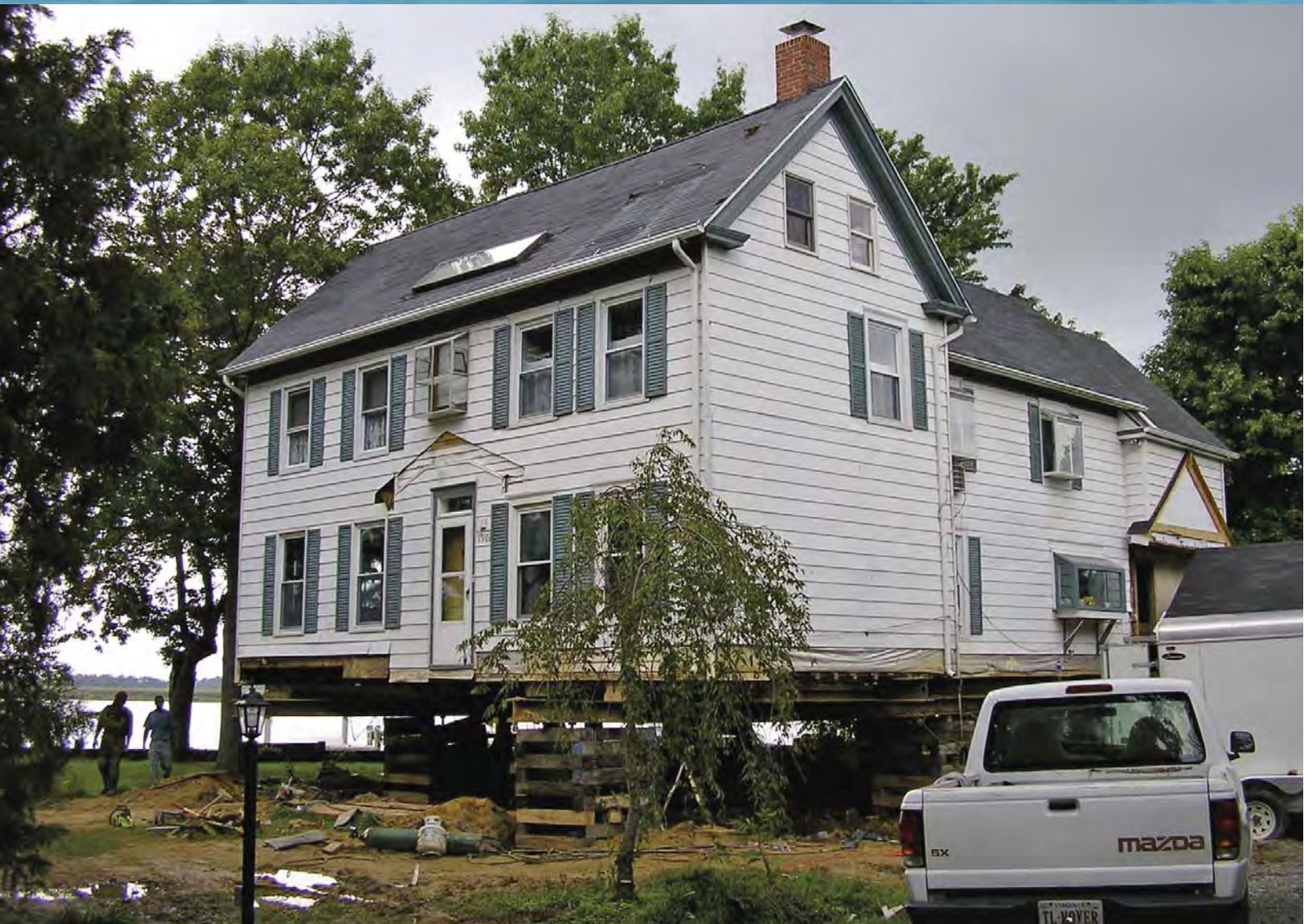
*Up and out of the floodplain, one painstaking inch at a time. Harriett and Bud Hankins added an additional four feet to the height of their house when they rebuilt after the devastating flooding of Hurricane Isabel. The process took nearly a year to complete. PHOTOGRAPH COURTESY OF HARRIETT AND BUD HANKINS.*
